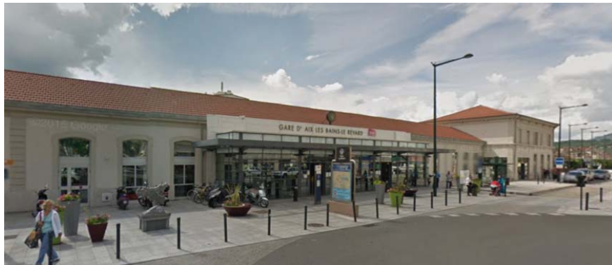
Photo 14: French National Railway Station, Aix-les-Bains
